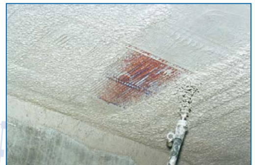
BEKA cooling ceiling as plaster ceiling
