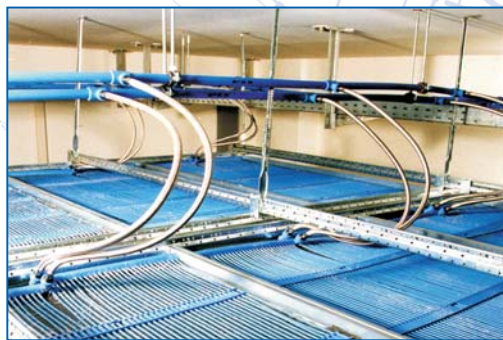
BEKA supply lines with quick-action couplings
