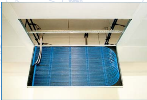
BEKA cooling ceiling as metal cassette ceiling
